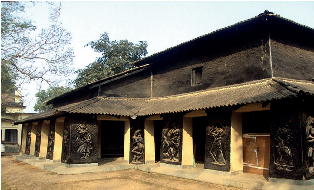
Fig. 9. Kalo Bari, a manifestation of vernacular architecture; courtesy & © Rabindra Bhavan Archives.
