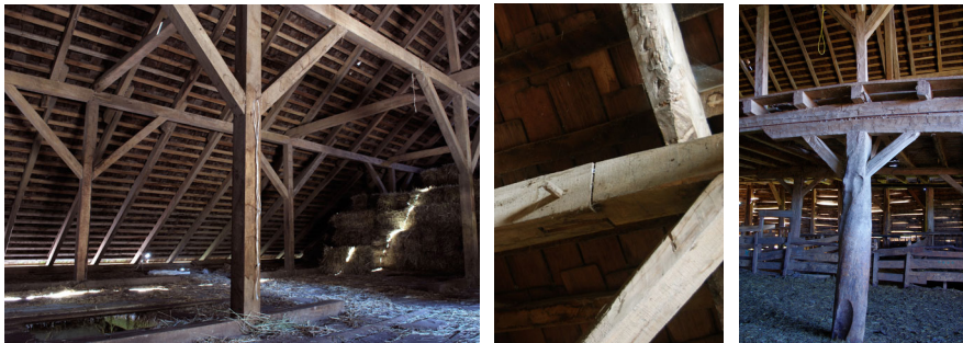
Fig. 144-145. Capannone Welman, Llanquihue; Fig. 146. Capannone Loebel, Puerto Octay
