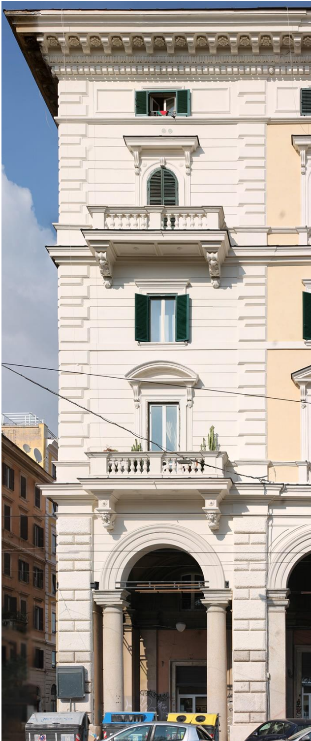
Fig.8: Rectified image of the corner bay of block XV (authors' elaboration).
