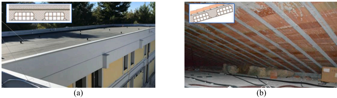
Fig. 5. Example of composite cast-in-place RC and masonry floor systems for (a) flat and (b) pitched roof.
