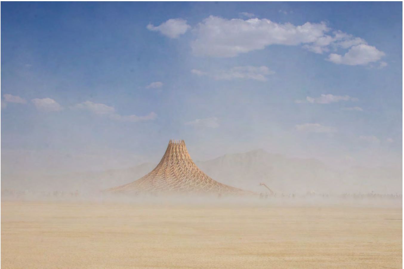
05. Galaxia Temple, progetto di Mamou-Mani Architects. Burning Man, 2018 | Galaxia Temple, design by Mamou-Mani Architects. Burning Man, 2018. Angus McIntyre
