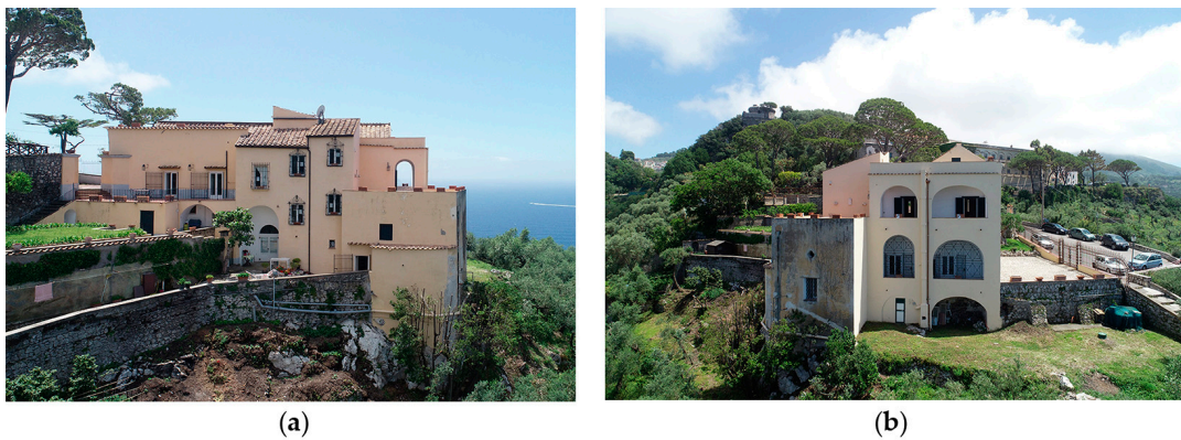
Figure 11. (a) Back elevation of the Villa. (b) North elevation with loggias and angular volume identified as pre-dating the rest of the building.
