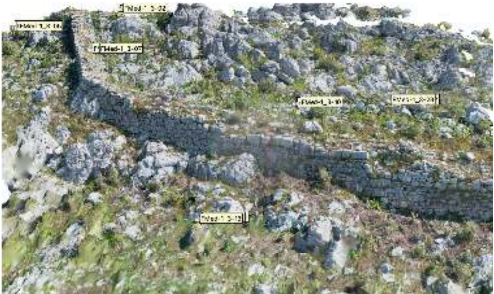
Figure 8 - A bird's eye view of a section of the Mediaeval fortifications from the digital 3D model, making use of oblique photographs
