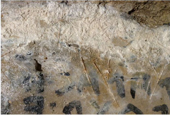
Figure 11. Atrium , carbonate depositions of different nature and typology are re-deposited on the pictorial layer.
