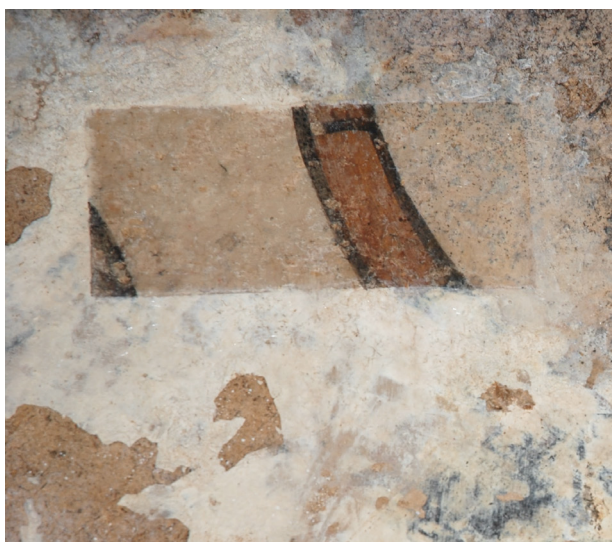
Figure 13. Detail of the biological patina of moonmilk, where it is thicker and harder, thereby protecting rather than damaging the murals.
