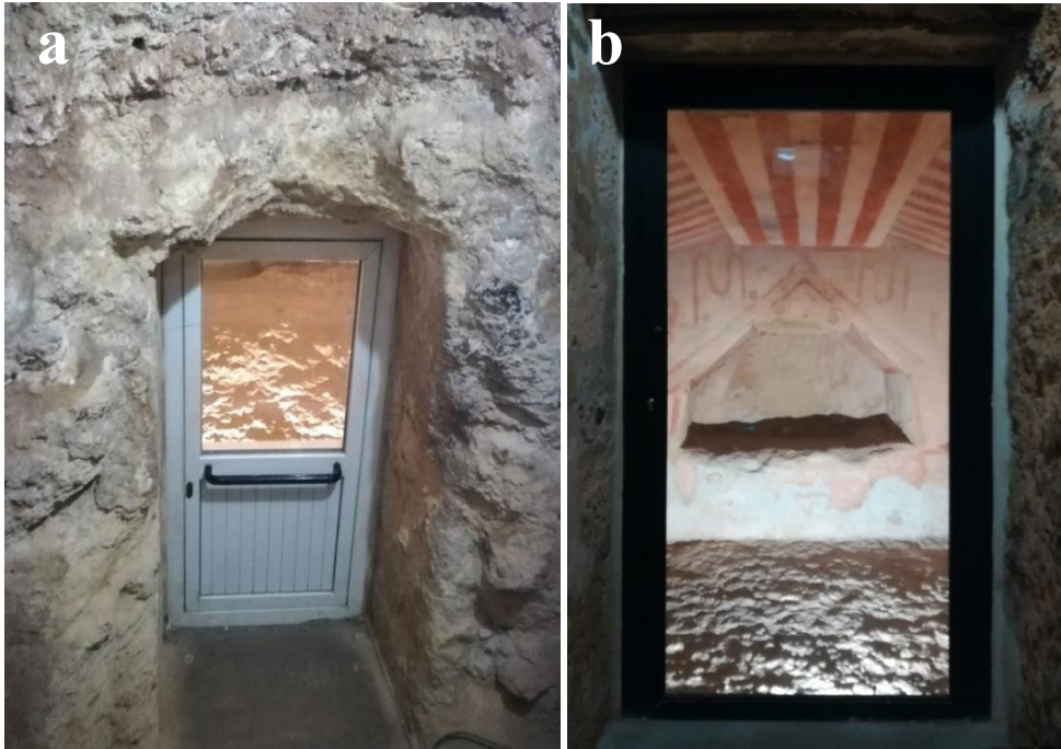
Figure 2. Examples of thermally insulating doors: earliest prototypes installed (a) most recent type (b): equipped with full glass.
