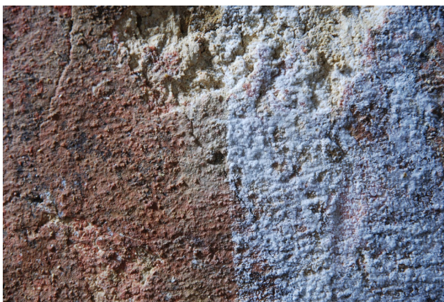
Figure 12. Detail of the wall where the biological white and powdery patina of moonmilk has been removed on the left side.
