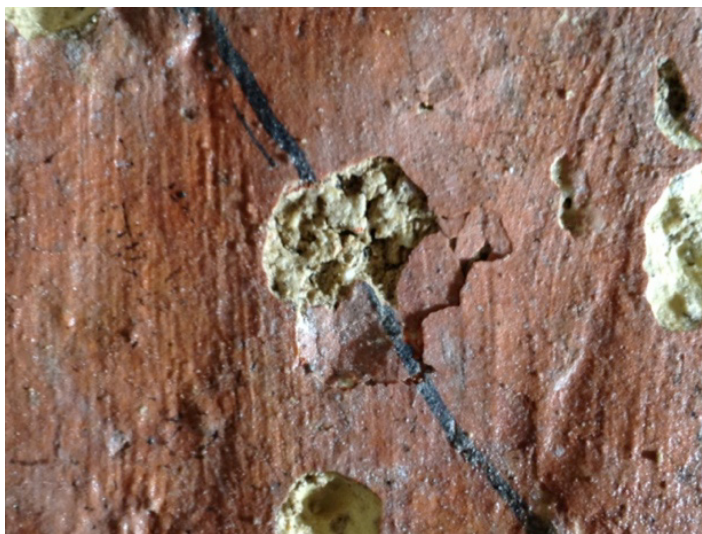
Figure 10. Atrium , voids of different sizes are present underneath the pictorial layer.
