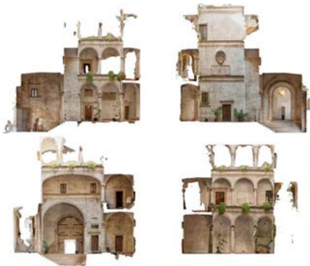
Figure 12. Rendering in orthographic projection of the four faces of the courtyard processed from the textured model
