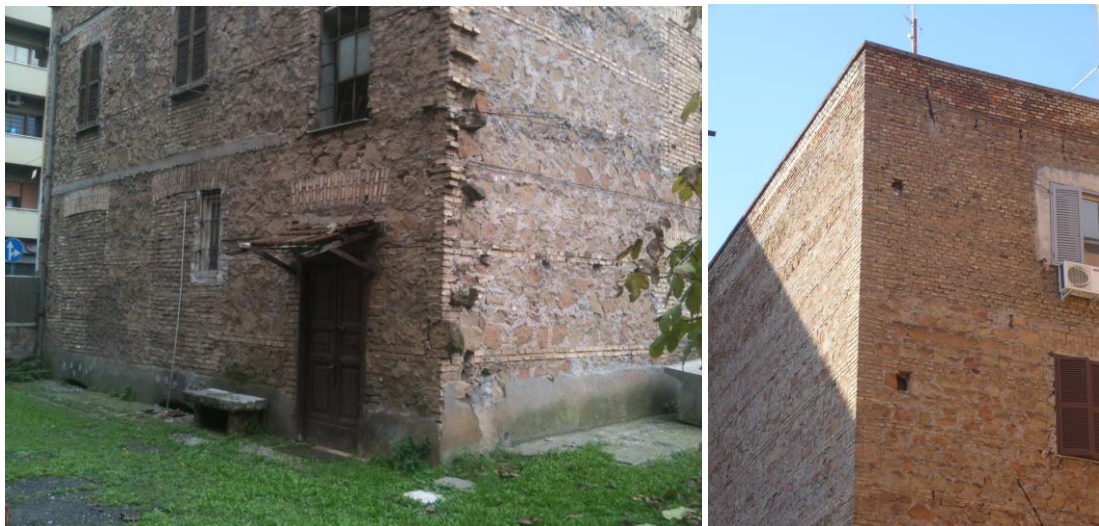
Figure 2: Walls typical of Rome between the mid-nineteenth and mid-twentieth centuries.
