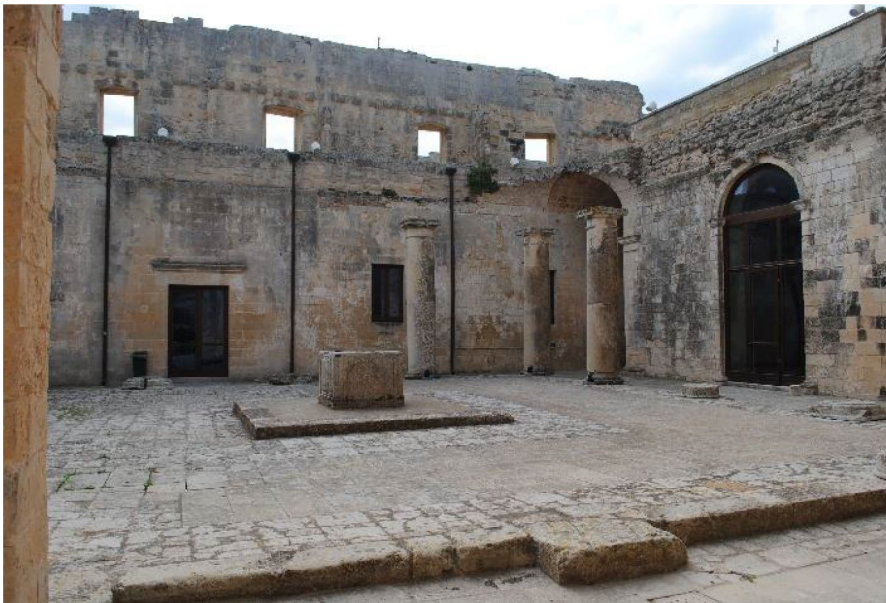
Fig. 3 The Augustinian church cloister: a glimpse of the interior of the cloister
