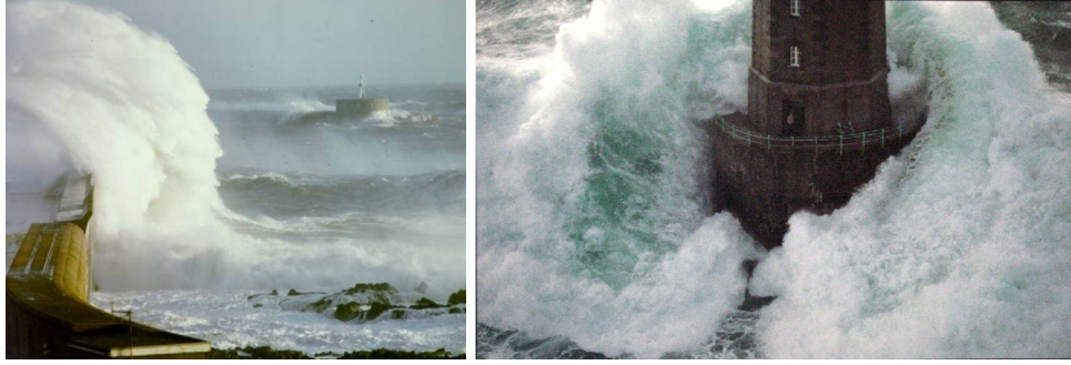
Figure 1.1.: Examples of water impacts on coastal structures under extreme sea states (Pictures taken from the web).
