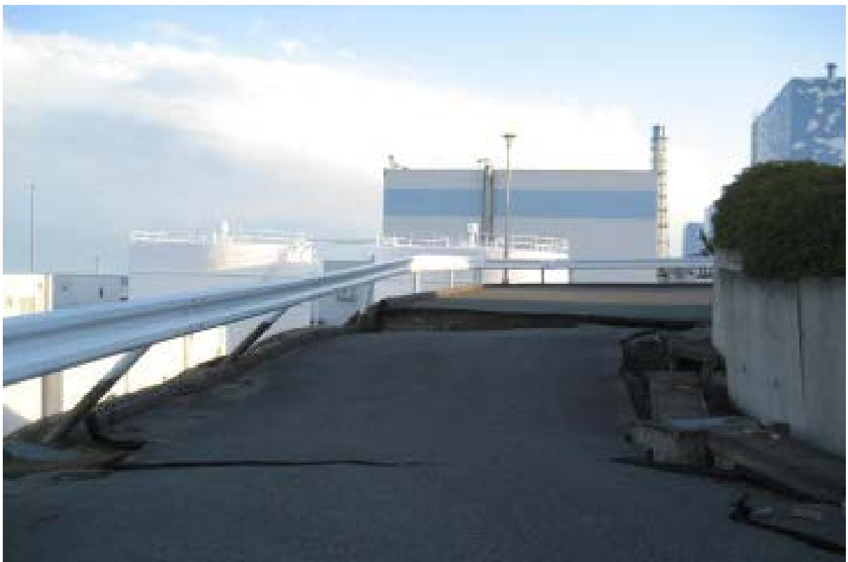
Figure 17. Street in the Fukushima Dai-ichi site
