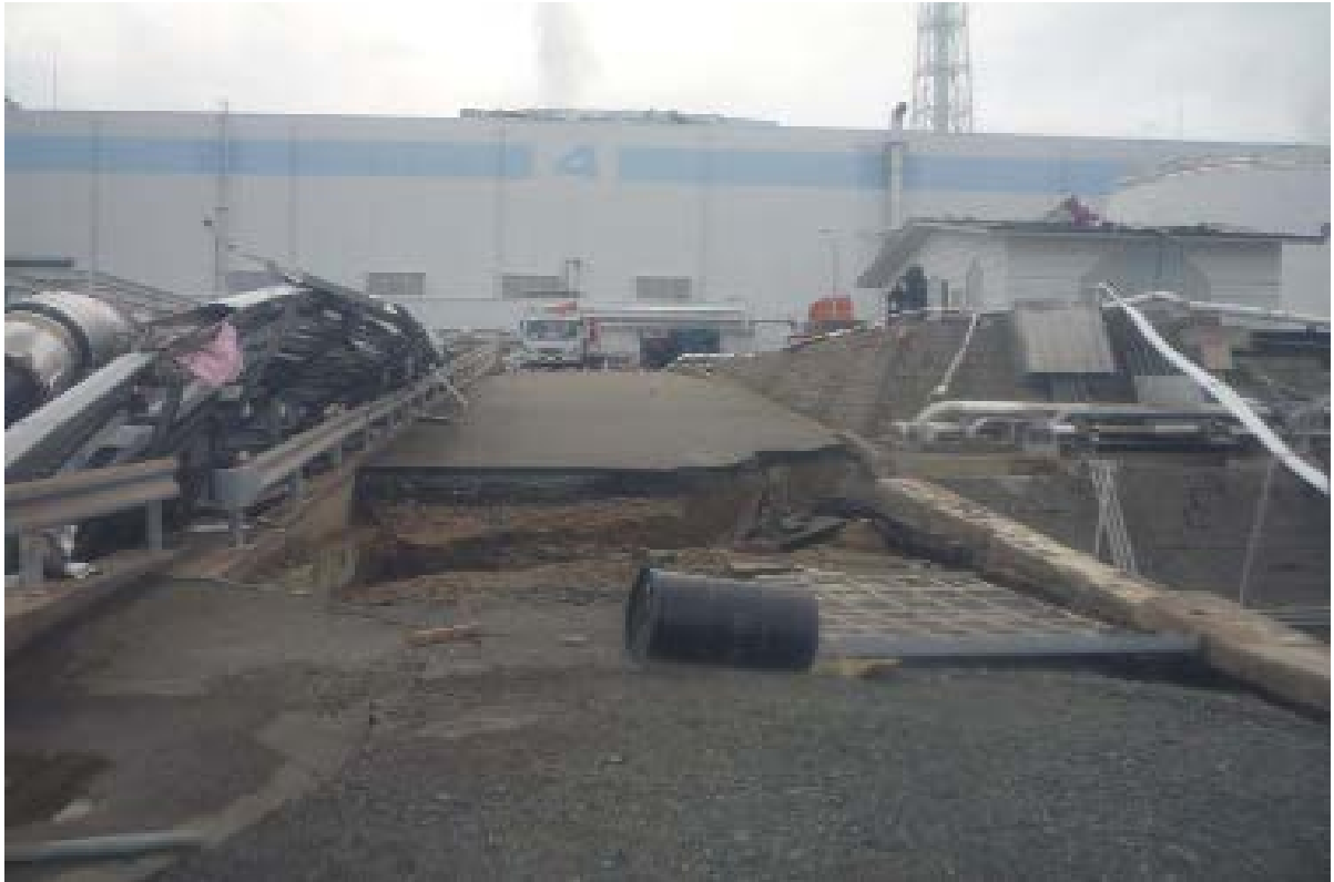
Figure 18. Street in the Fukushima Dai-ichi site
