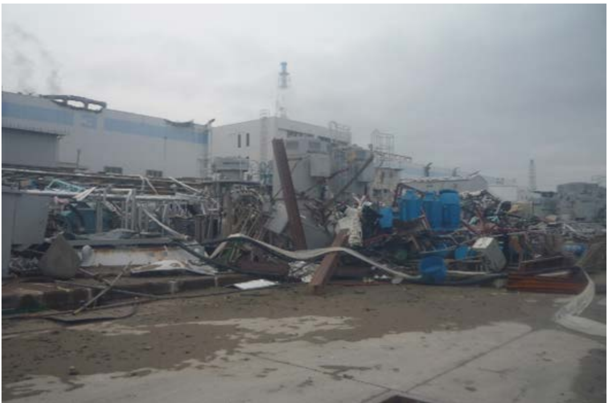
Figure 19. Debris after the tsunami in the Fukushima Dai-ichi site
