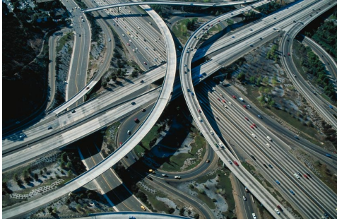
(a) Clothoids curves are often used in high-ways design
