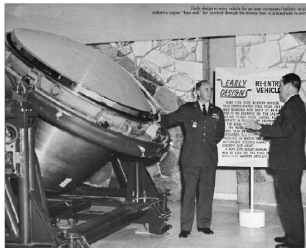
Figure 2: The copper heat sink of the intercontinental ballistic missile (ICBM).
