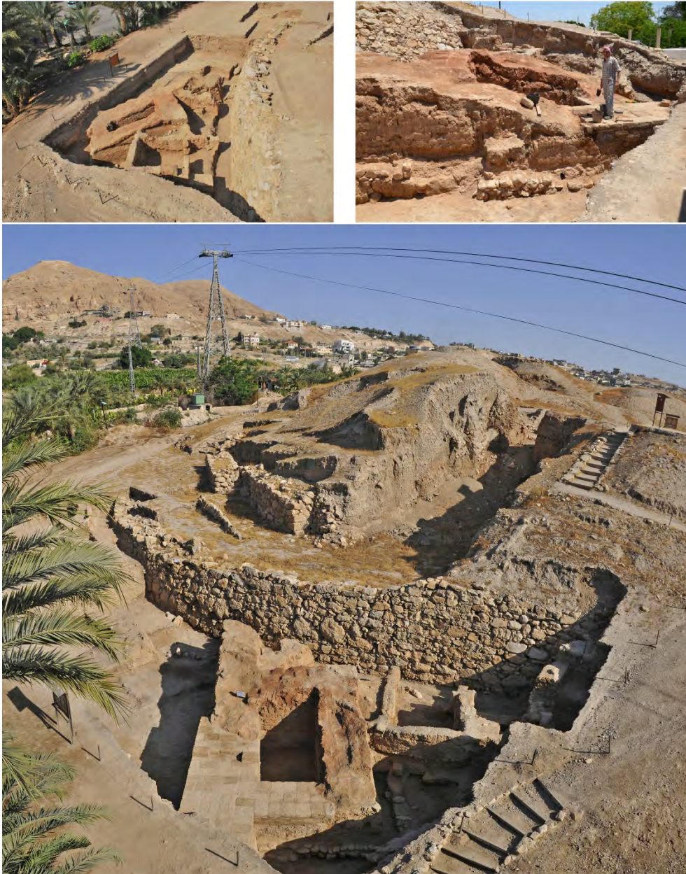
Fig. 14 - Tower A1 before, during and after restoration works.
