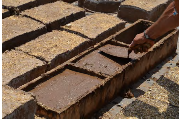
Fig. 15 - Making of mud bricks to be used in the restoration of Palace G.
