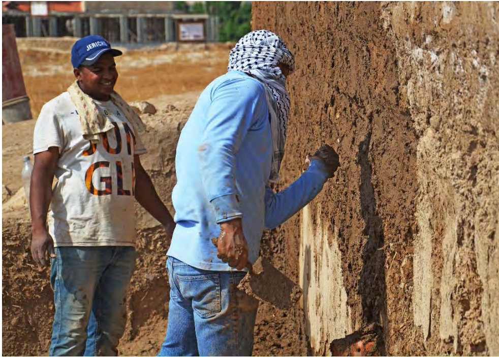
Fig. 23 - Specialized workers coating a mud bricks wall with traditional plaster.
