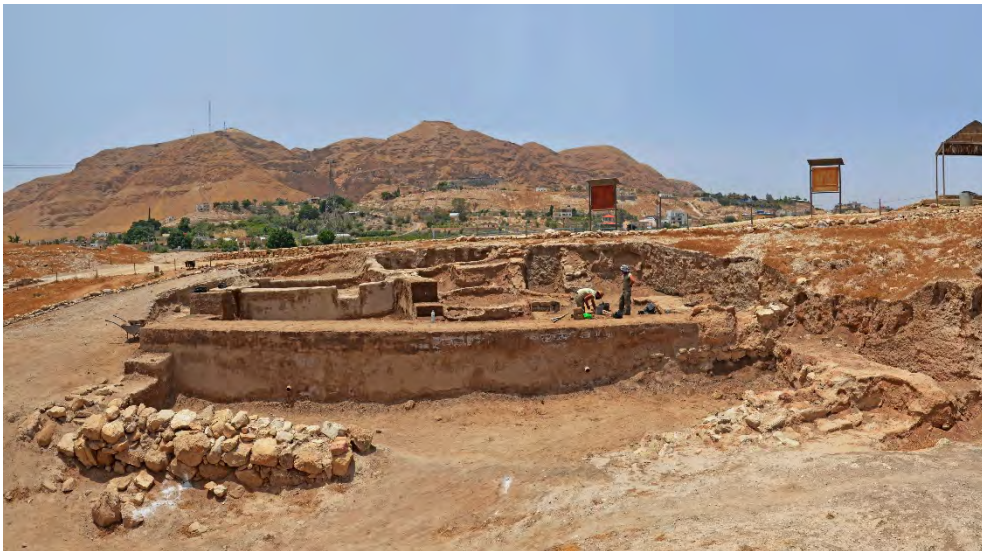
Fig. 20 - General view of Palace G after restoration works.
