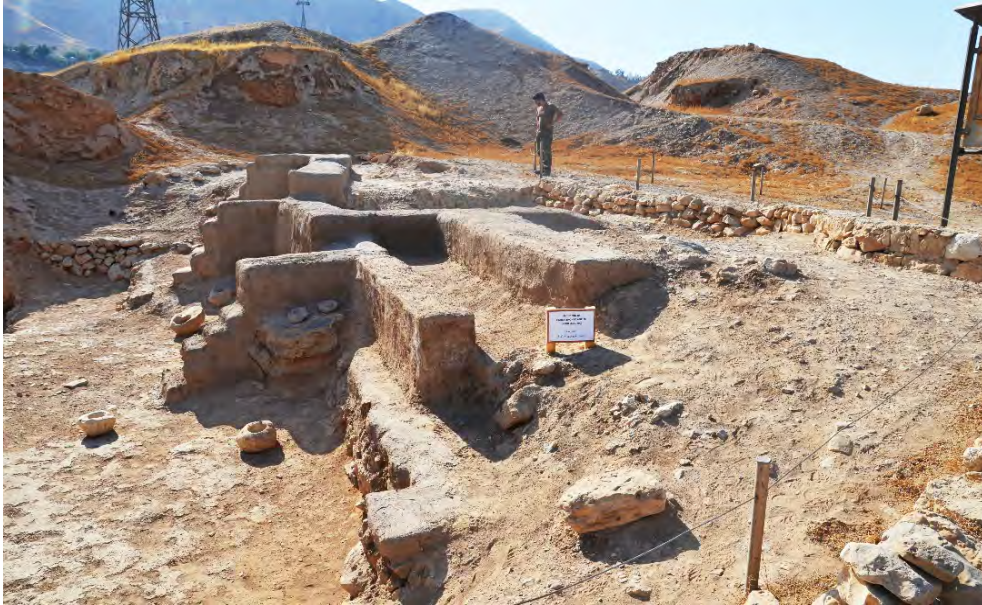
Fig. 25 - General view of Building B1 after rehabilitation with signal indicating name and dating of the monument.
