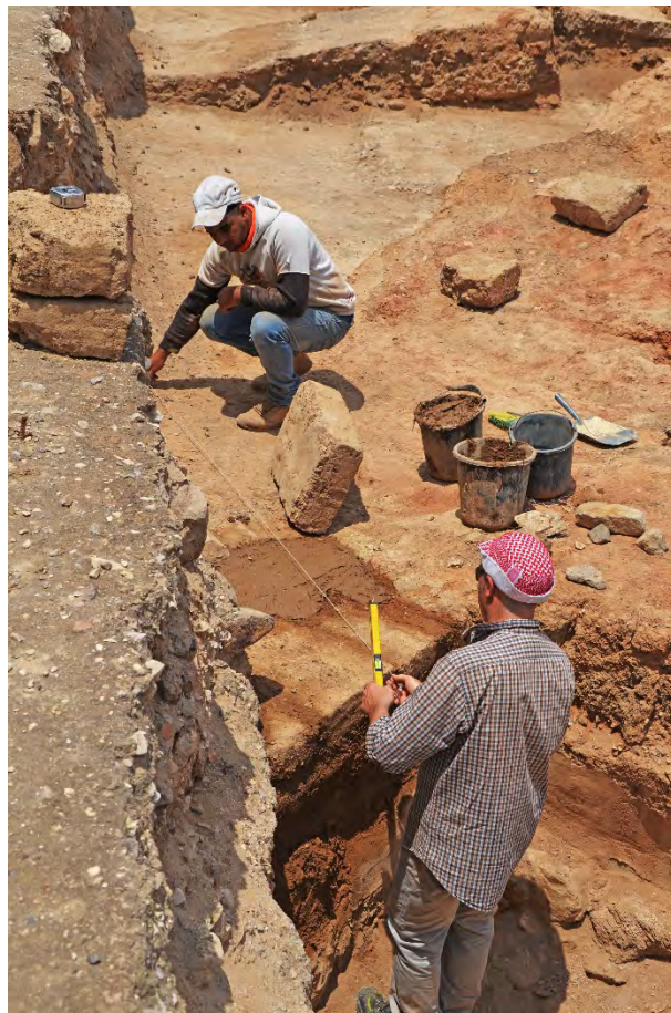
Fig.16 - Restorers preparing the mortar bed for the sacrifice layer of new bricks.
