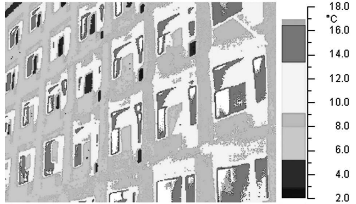
Figure 2. Thermographic survey: building main facade.
