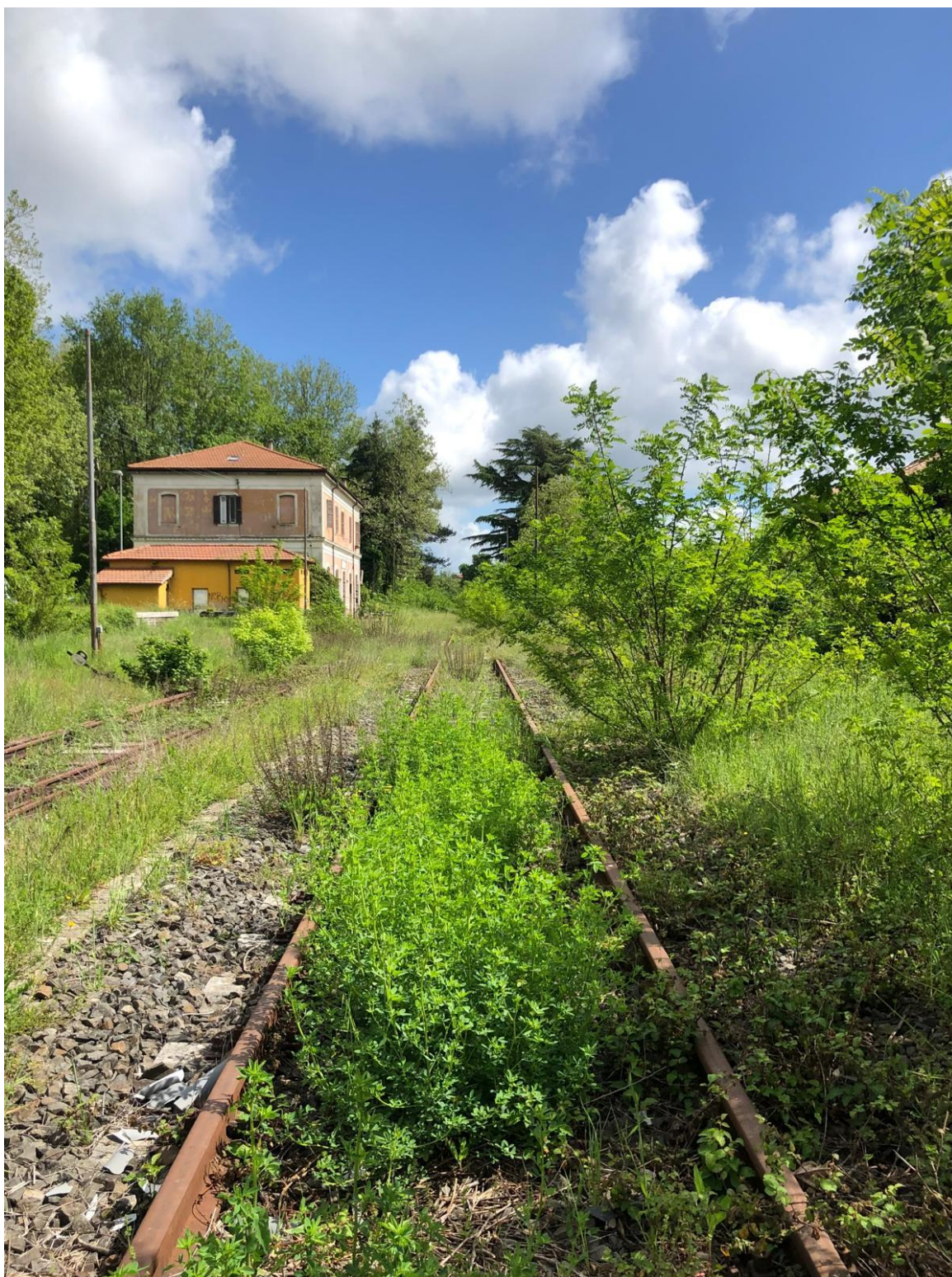
Fig. 1 - Civitavecchia - Capranica - Orte railway line (source: author's photo)
