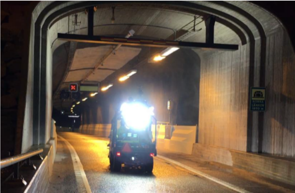
Fig. 5.5: Mobile mapping system for tunnel data acquisition
