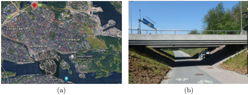
Fig. 5.8: Bridge test site
