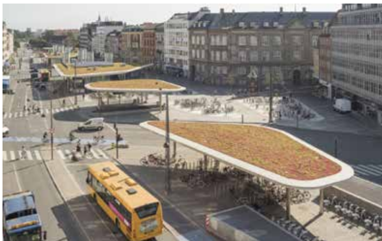
Fig.3.0.2 COBE + Gottlieb Paludan Architects, Nørreport Station, Copenhagen, Danimarca.
