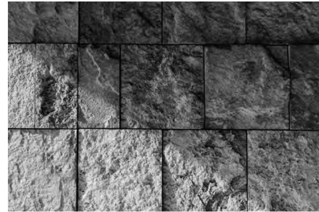
FIGURE 5 Travertine's rough texture resulting from the guillotining in Getty Foundation Project's exterior, by Richard Meier, photo CC: Wil Stewart
