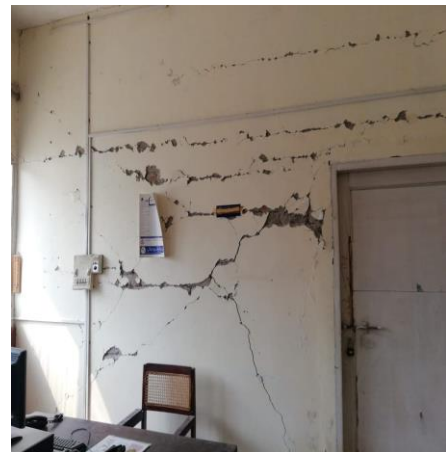
Figure 5. Cracks and damages observed in the infill walls in different parts of the building
