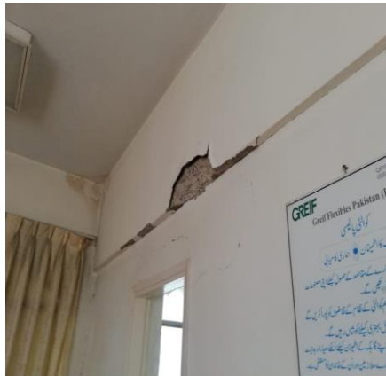
Figure 4. Cracks observed in column and infill (left), and joints (right)
