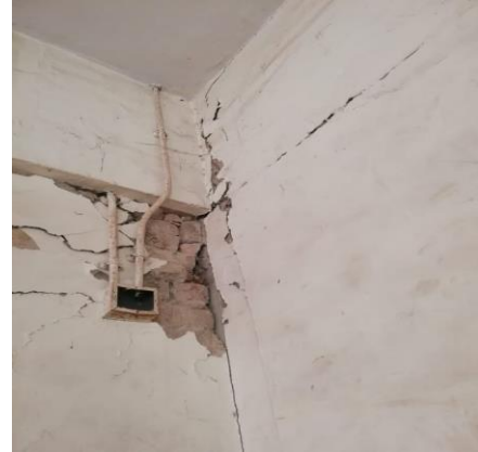
Figure 4. Cracks observed in column and infill (left), and joints (right)
