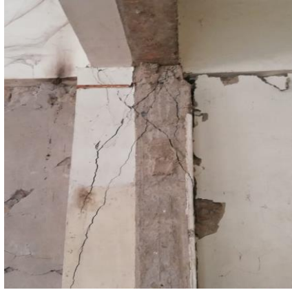
Figure 3. Cracks observed in beam (left), and column (right)
