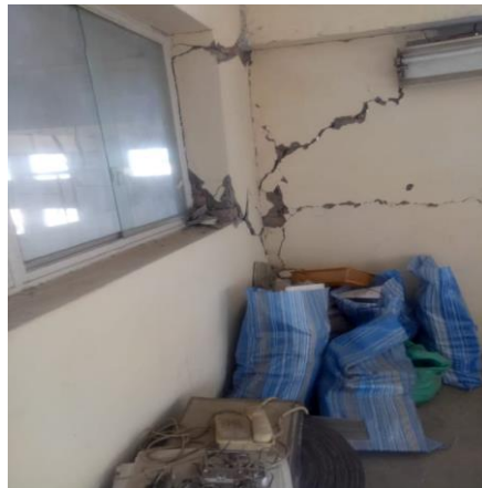
Figure 5. Cracks and damages observed in the infill walls in different parts of the building
