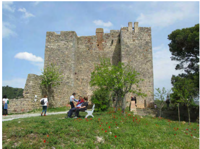
8.3/ The south facade of the Fortress of Talamone.
