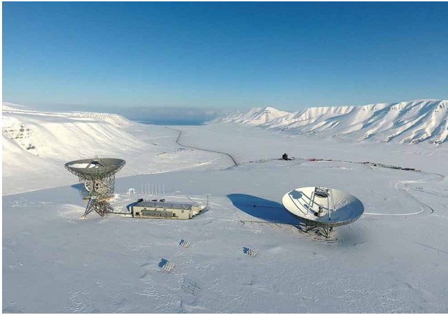
1.17/ EISCAT Svalbard Radar (ESR) near Longyearbyen, Spitzbergen Island, Svalbard Archipelago, Norway. The site is located above the Arctic Circle and is close to the North Pole. The facility has two antennas: a 32-metre mechanically fully steerable parabolic dish antenna and a fixed parabolic antenna, aligned along the direction of the local geomagnetic field. The sensors are computer-controlled, but can be controlled by the other facilities of the European Incoherent Scatter Scientific Association (EISCAT). Source: European Incoherent Scatter Scientific Association, 2016. Fotografia di Craig Heinselman.
