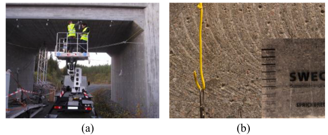
Fig. 1. Visual inspection (a) using graduated cards (b).
