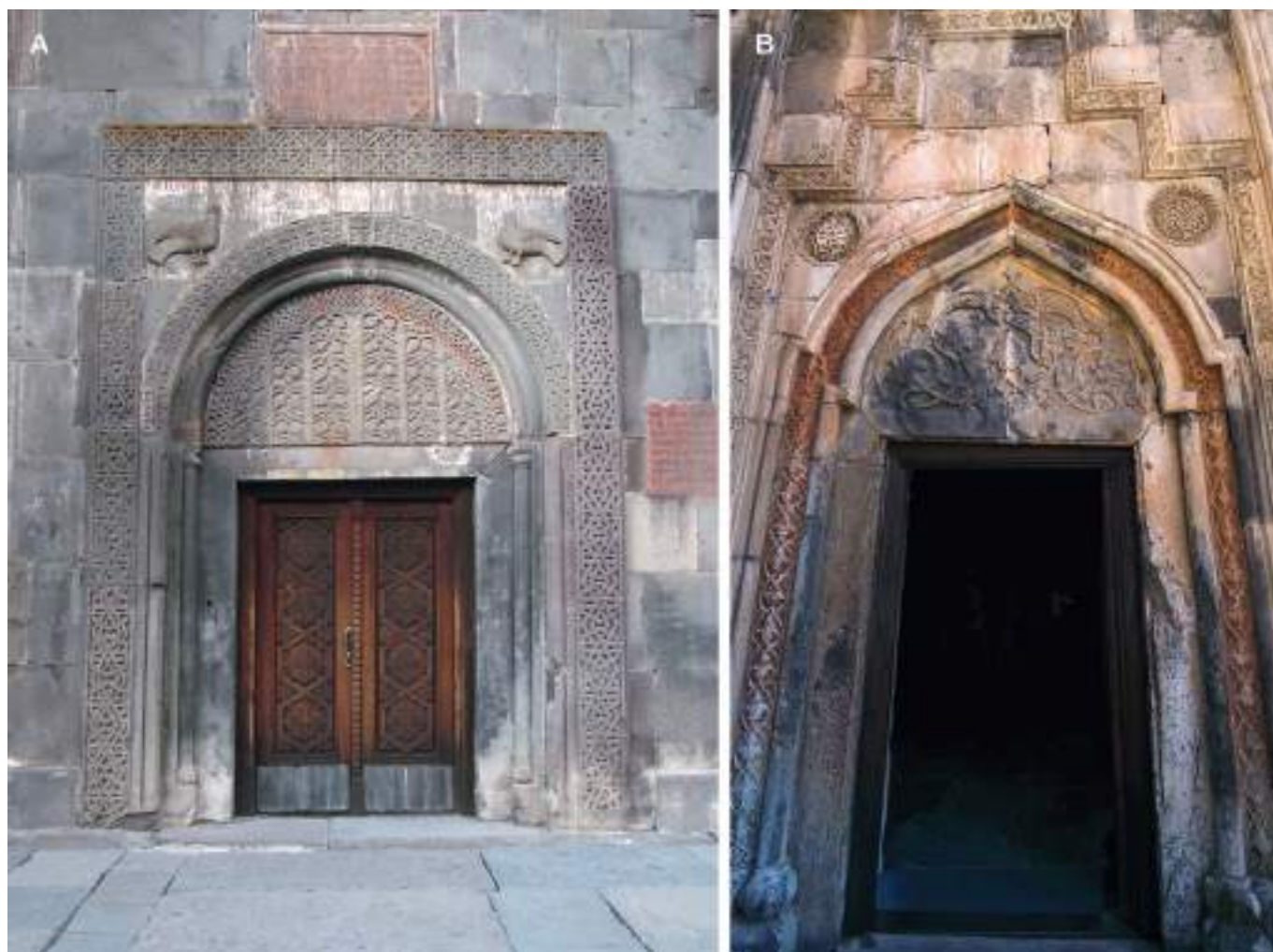
Fig. 3 – A) Southern portal; B) Western portal (photo R. Zanone).
