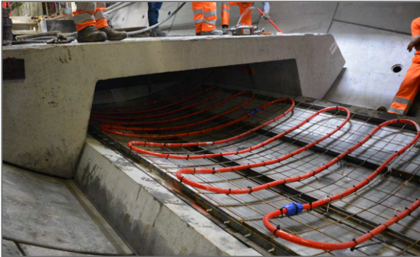
Figure 4: Installation of Smart Flowing during TBM advancement.
