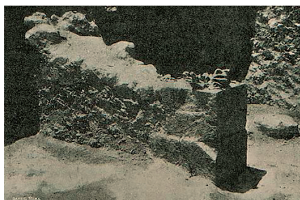
Fig. 2 : Walls and column-base of the later “Mycenaean” phase (Pernier 1904, 322)
