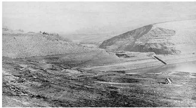
Figure 2.3 The ruptured embankment viewed from inside the reservoir of Dale Dyke dam, few days after the disaster (Photo source: www.mick-armitage.staff.shef.ac.uk/sheffield/photogal/picflud1.html )
