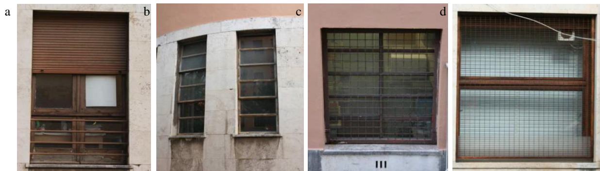
Figure 3. (a) Original wooden window; (b) original iron window; (c) modern PVC window; (d) modern aluminium window.
