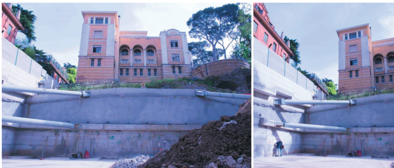
Figure 10. Excavation of the atrium and installation of the steel struts.
