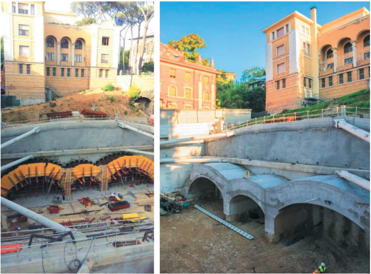
Figure 16. Construction of the reinforced concrete entrance portal.
