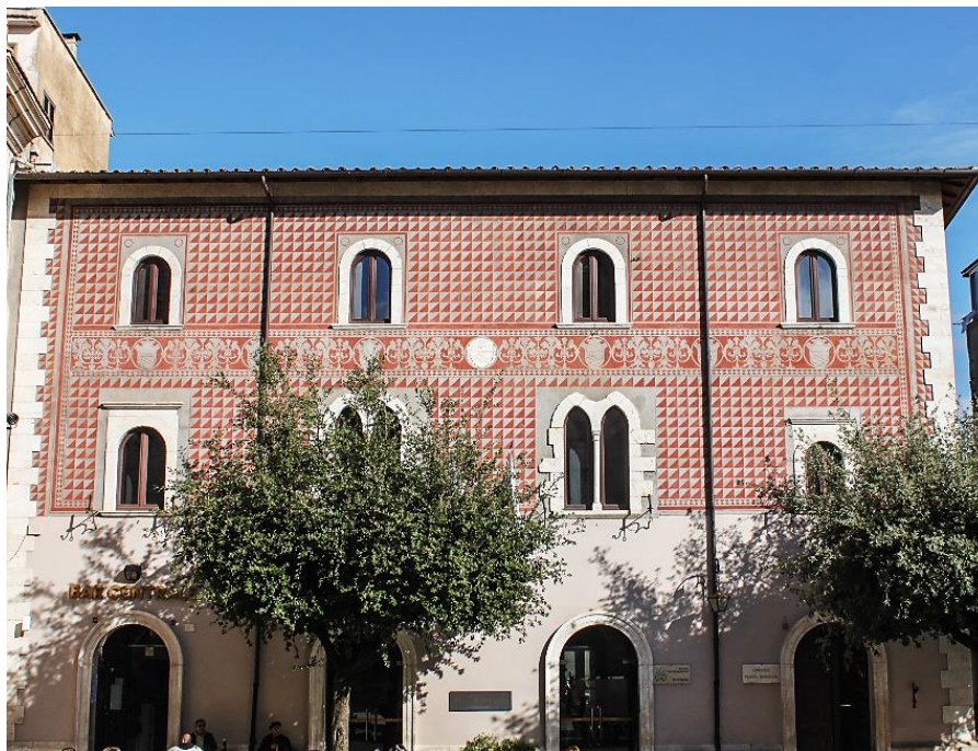
Figure 2 The Archaeological Museum of Privernum (Latina, Italy): the main entrance (second door from left at the ground floor), the double-arched windows (first floor) and the façade in Renaissance style with an amaranth and lead-grey graffito decoration.
