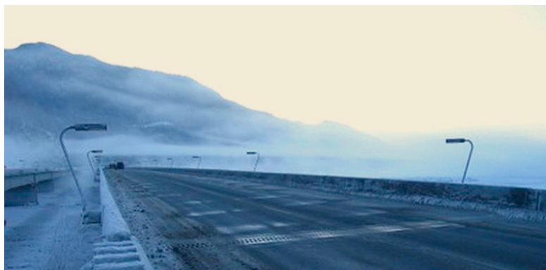
Figure 4. Example of Fixed Automated Spray Technology Systems (FAST) [54].
