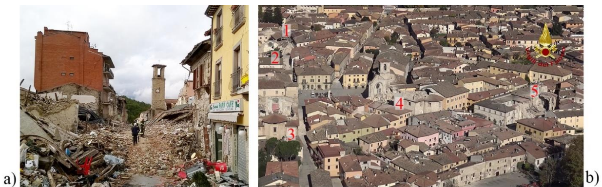
Figure 2. a) Amatrice, after the August 24 th event. Extensive damage and collapses in ordinary unreinforced masonry buildings and damage without collapses in tall buildings: six-storey reinforced concrete building, on the left, and Clock Tower from Corso Umberto I. b) Part of the historical centre of Norcia after the October 30 th event in the snapshot of a movie released by the Corps of Firefighters ( www.vigilfuoco.tv ). Limited damage to ordinary unreinforced masonry buildings and extensive collapses to churches: 1) Santa Rita, 2) San Francesco, 3) Santa Maria Argentea, 4) San Benedetto, 5) San Filippo.
