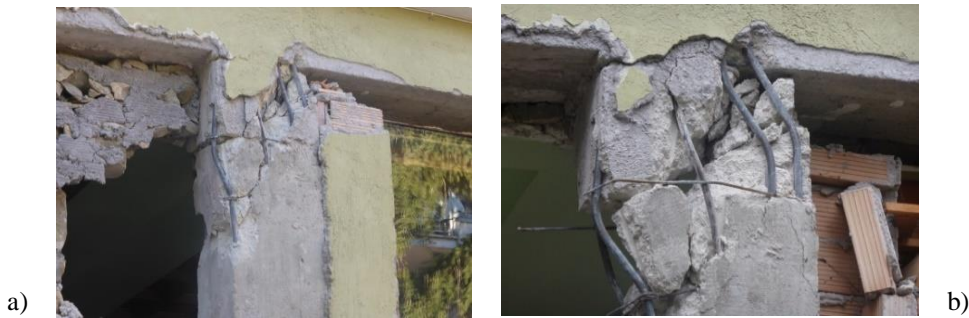
Figure 14. Progressive damage to a reinforced concrete building in Amatrice: a) after the August 24 th event; b) after the October 30 th event.
