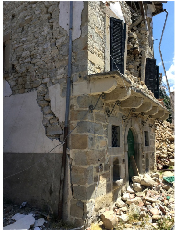
Fig. 14. Reduced strength of lateral walls compared to large-units wall intersections, Amatrice, Retrosi.
