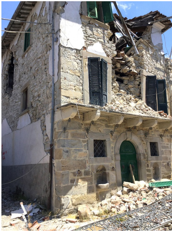
Fig. 14. Reduced strength of lateral walls compared to large-units wall intersections, Amatrice, Retrosi.
