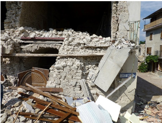
Fig. 6. a) I-beam and hollow clay block floor, Amatrice, Retrosi; b) Precast reinforced concrete beams and hollow clay block floor, Amatrice, Moletano.
