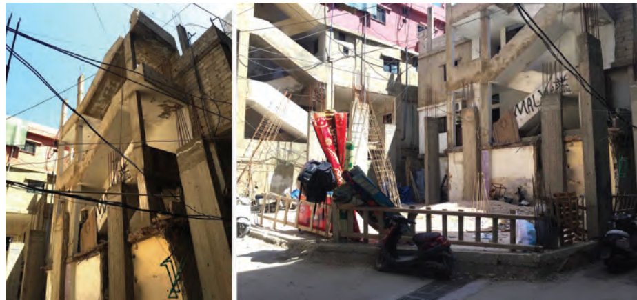
Fig.14) The chaotic structural systems (left). Foundation of new buildings start from above ground (right).
