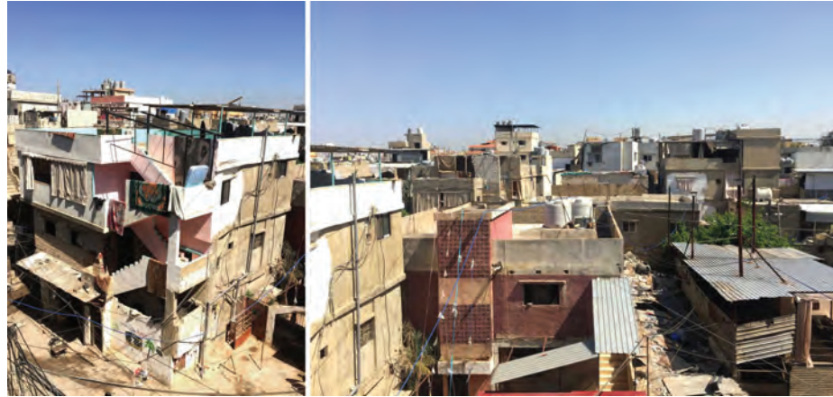
Fig. 13) The building typology. Buildings grow vertically in order to cater for the needs of inhabitants.
