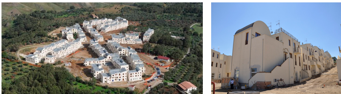
Figure 6. The new town of Cavallerizzo di Cerzeto (Calabria, Italy) destroyed by a landslide in 2005 and constructed in a nearby area (photos by the website of Italian Civil Protection).
